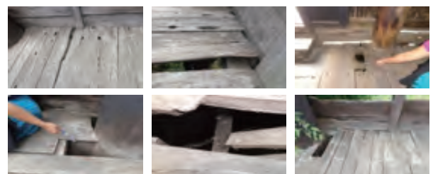
Figure 21 Damages assessment on floorboards
