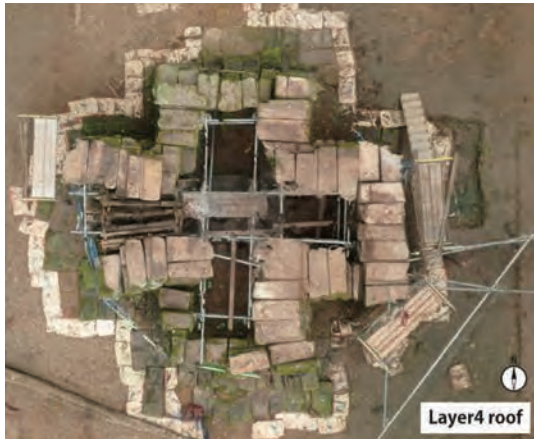
East Gate of the Ta Nei temple during the dismantling process
