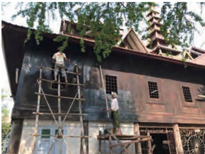
Figure 32 Applying traditional treatment on exterior wall
